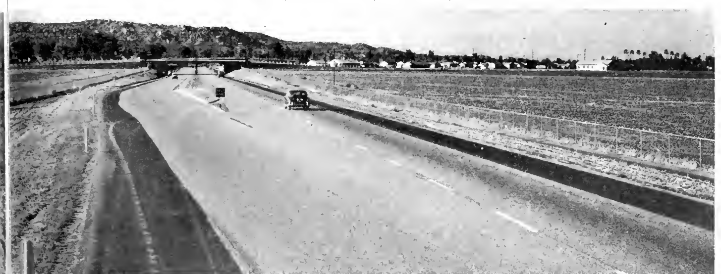
Looking north at the transition from two lanes to four lanes divided. The four-lane divided highway is continuous from this point on the Perris Bypass into the City of Riverside.
